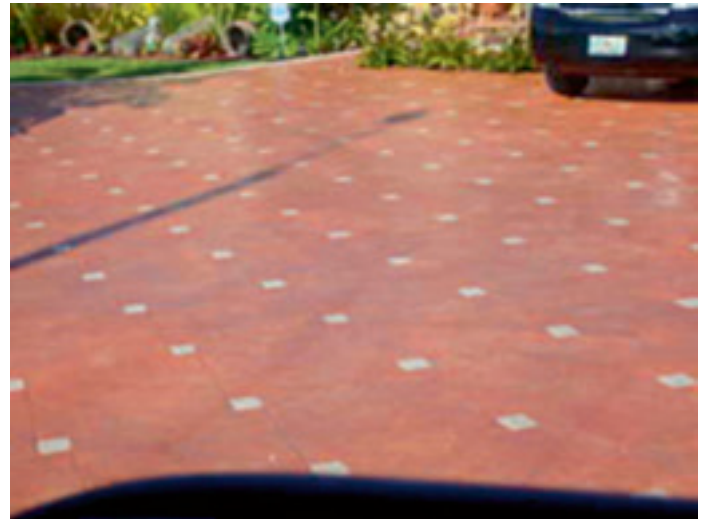
MIAMI, Fla. - Intricately designed, patterned and art-deco driveways are highly prized by Miami-Dade homeowners. In order to save them, the water department threads the much-needed new 2-inch HDPE water pipe-line under the pavement and yards, which also saved time and labor costs.
